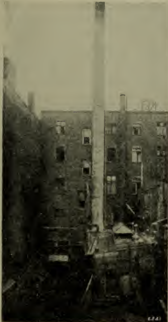
COATING A CHIMNEY 120 FT. HIGH AT THE CENTRAL HOTEL, BERLIN.
